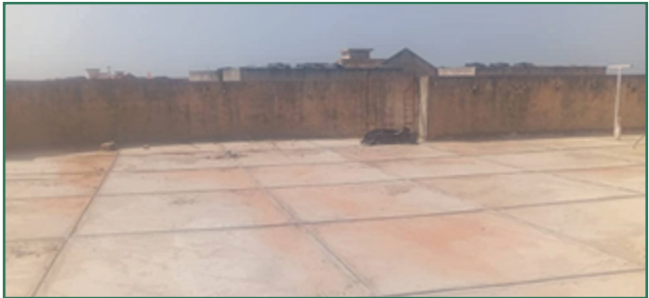
Roof floor washed terrazzo preparation
