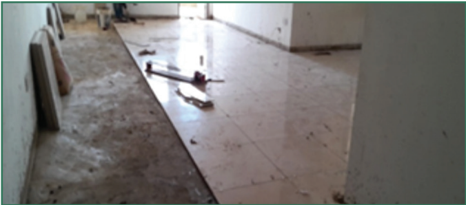
Floor tiling of rooms in Block 13
